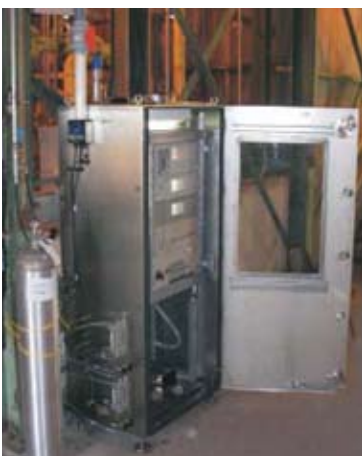
MMS Mercury Monitoring System installed at a hydrogen plant
